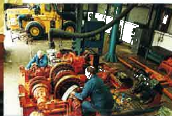
IHI CCH250 undergoing refurbishment.
