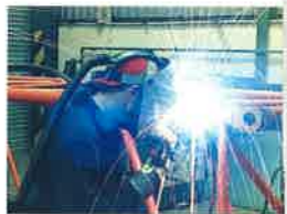
Crane boom repairs being undertaken in our fabrication shop.
