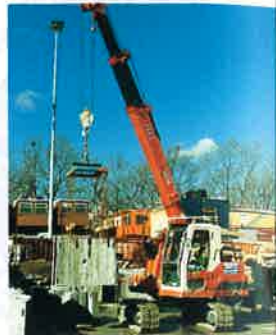
IHI CCH50T working on the Jubilee line extension in London.
