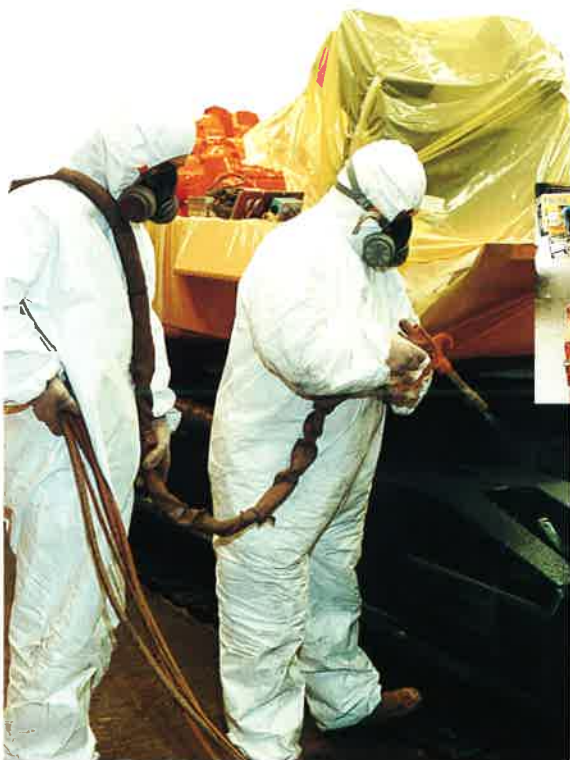
Latest technology airless hot spray equipment in use in our paintshop.
