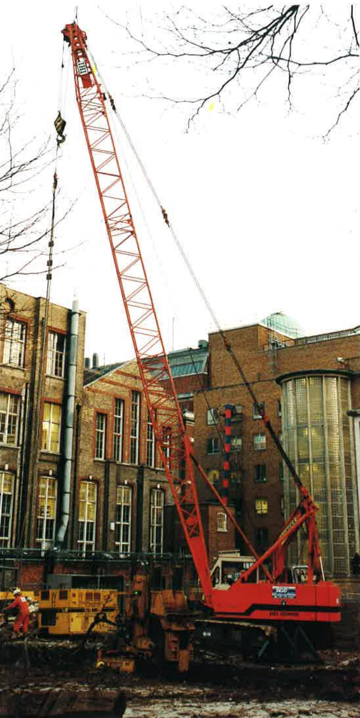
IHI CCH400 on a piling contract for Stent Foundations.
