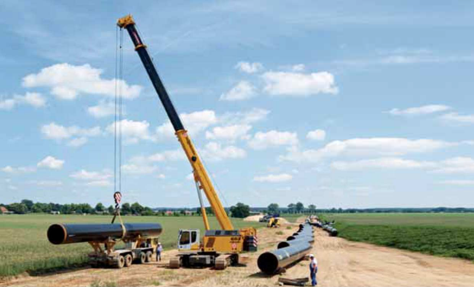
683 R - Installation of large pipes; Germany 683 R - Installation großer Rohre; Deutschland
